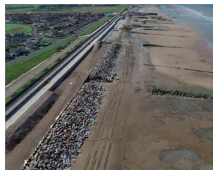
Completed section of lower rock revetment [Image: Wyre Council]
